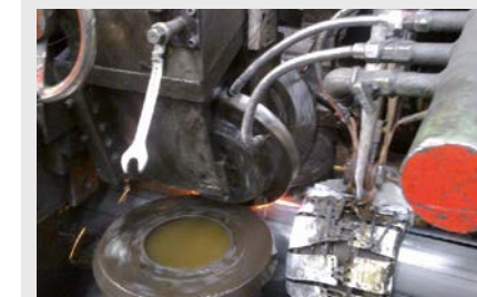
Temperature monitoring of pipe rims shortly before welding
