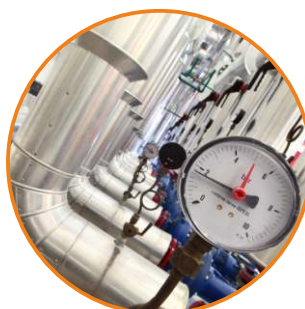
Heat exchange unit www.pedak.nl
