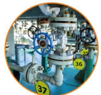
Water treatment plant
