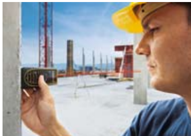
Measuring long distances thanks to Power Range Technology™ from Leica Geosystems.
